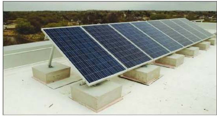
The roof of Enermodal Engineering's new building, "A Grandeur View," features 5.5 kW of photovoltaics (PVs). Under LEED 1.0, this system received one point whereas the same system would receive three points under LEED 2009.
